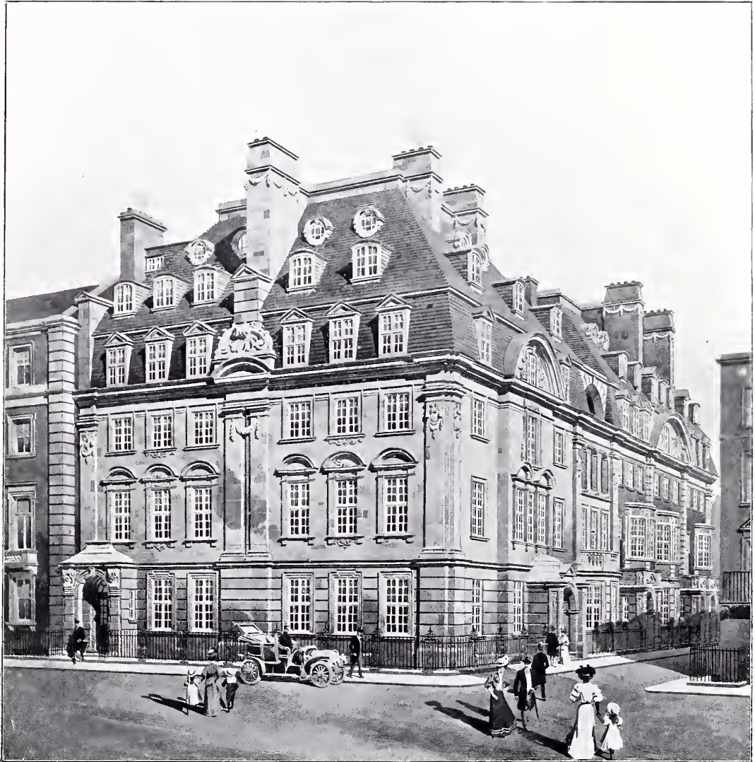
1503. Rebuilding in Upper Grosvenor Street, Mayfair, W. D. CARÖE, Architect. Building Owners: Higgs and Hill, Ltd., Crown Works, South Lambeth Road, S.W.
